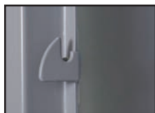
Main door latch hooks welded to frame
